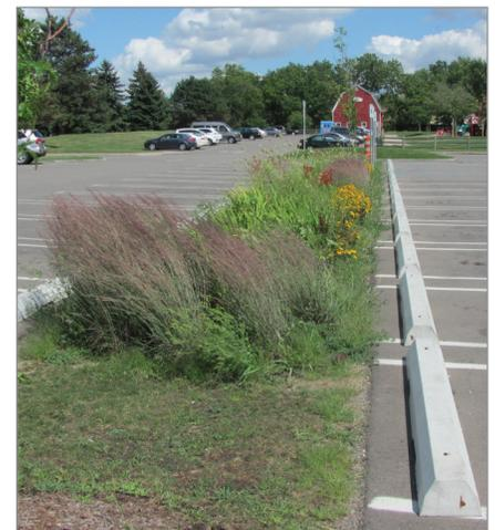
*An existing parking lot in Southfield, Michigan, was restriped and a section of pavement at the low point was removed and planted for stormwater management*
