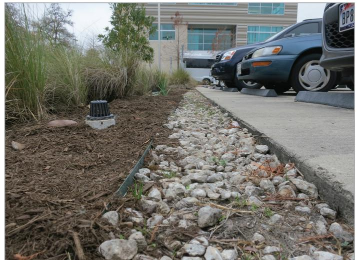
*Stone infiltration trench installed around the outside perimeter of an existing parking area to manage the runoff from the parking area.*
